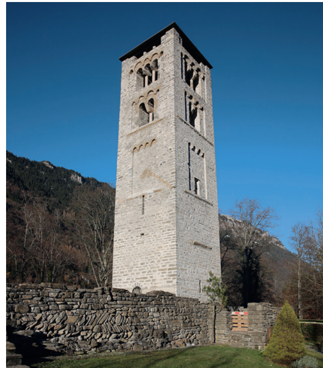
The bell tower, which now stands at a height of 16 m, originally had another belfry-stage with triforia and a pyramid roof.
