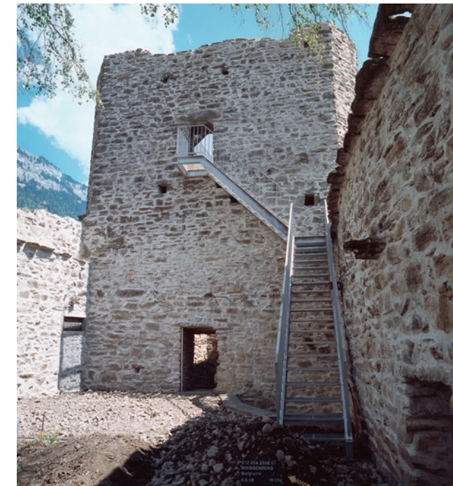
Castle courtyard with the façade of the east tower. The old steps were replaced by metal stairs leading to the elevated entrance into the ceremonial hall. The ground-level entrance is a post-medieval addition.
