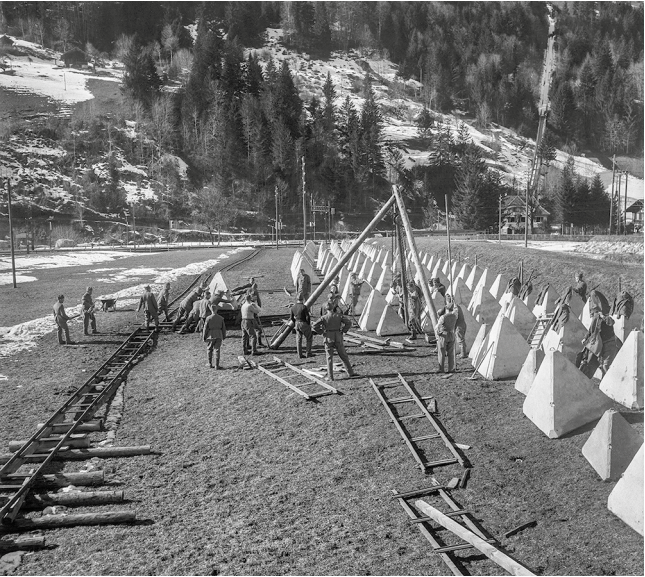
Construction of dragon's teeth in 1941 during the Second World War.
